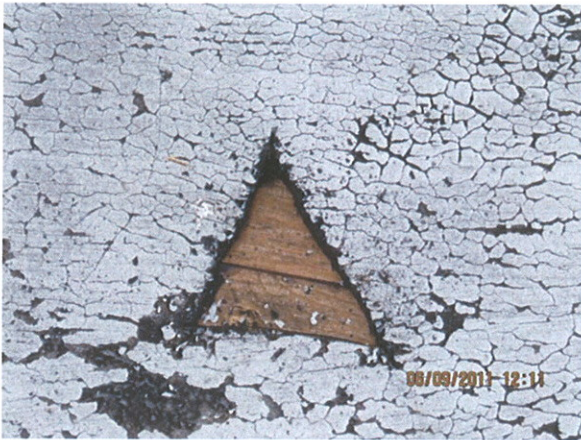
Sample 721-2 Middle of Roof
