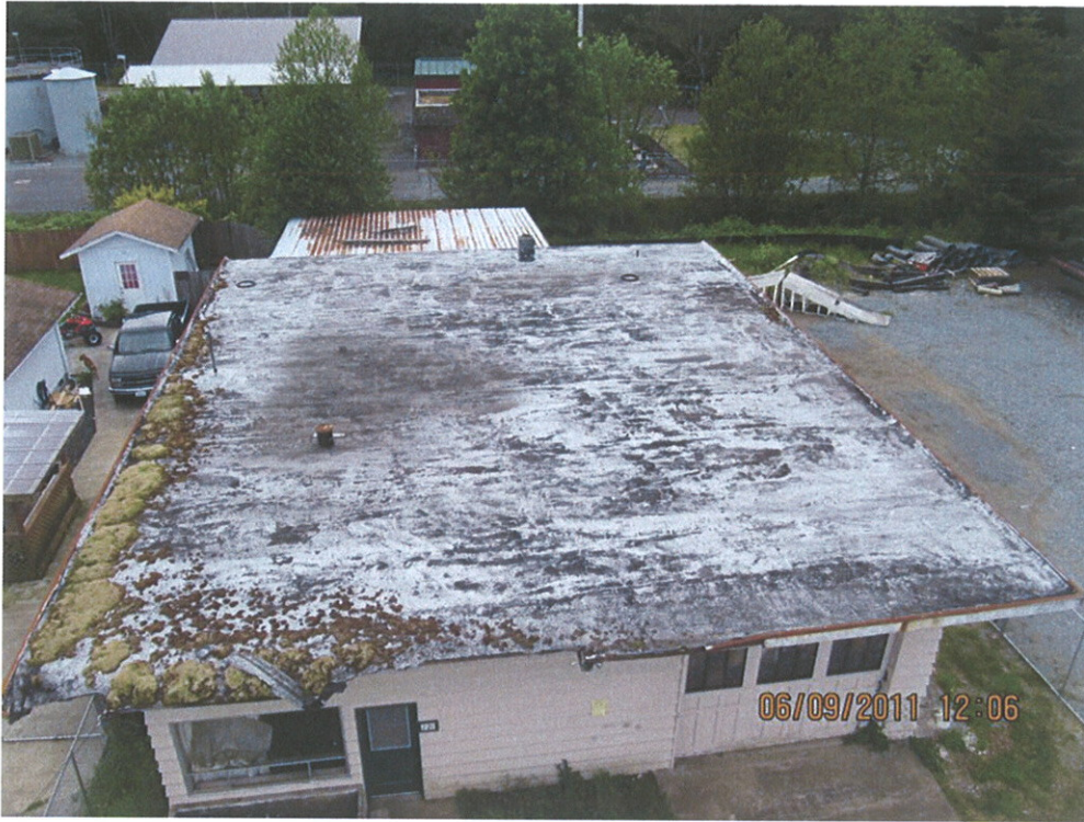
721 Simpson, McCleary, WA (Float Shed)
