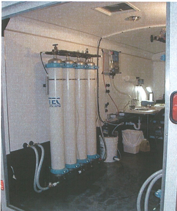
The picture on the left shows one set of filters. Source water enters through the hose inlet in the wall, passes through a flow meter, past a chlorine injection point, through an in-line static mixer, into the inlet manifold, down through the filter media. Product water is discharged through the wall. The pail holding the sodium hypochlorite solution can be seen to the right of the filter vessels and the in-line chlorine analyzer is on the wall above the NaOCl container. The sample ports and analytical equipment is forward of the chlorine analyzer. A second container of Ferric Chloride solution and feed pump is provided for pilot testing for arsenic removal.
