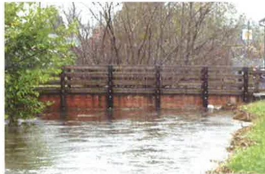
Sam's Canal; Water hitting pedestrian bridge
