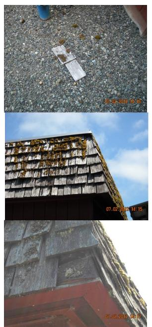
We have received three quotes for to remove the existing shake roof and replace it with new snap lock metal panels (similar to the other buildings on the property and the fire department roof). The quotes are as follows:
