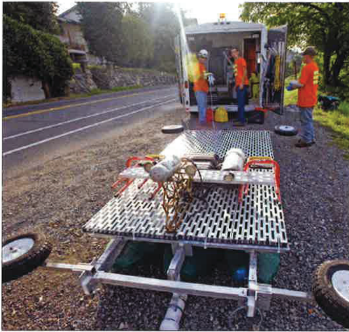
A crew from Pipe Experts Inc. of Tumwater, Wash., prepares a CCTV camera and sonar platform for the inspection of a 96-inch interceptor.
