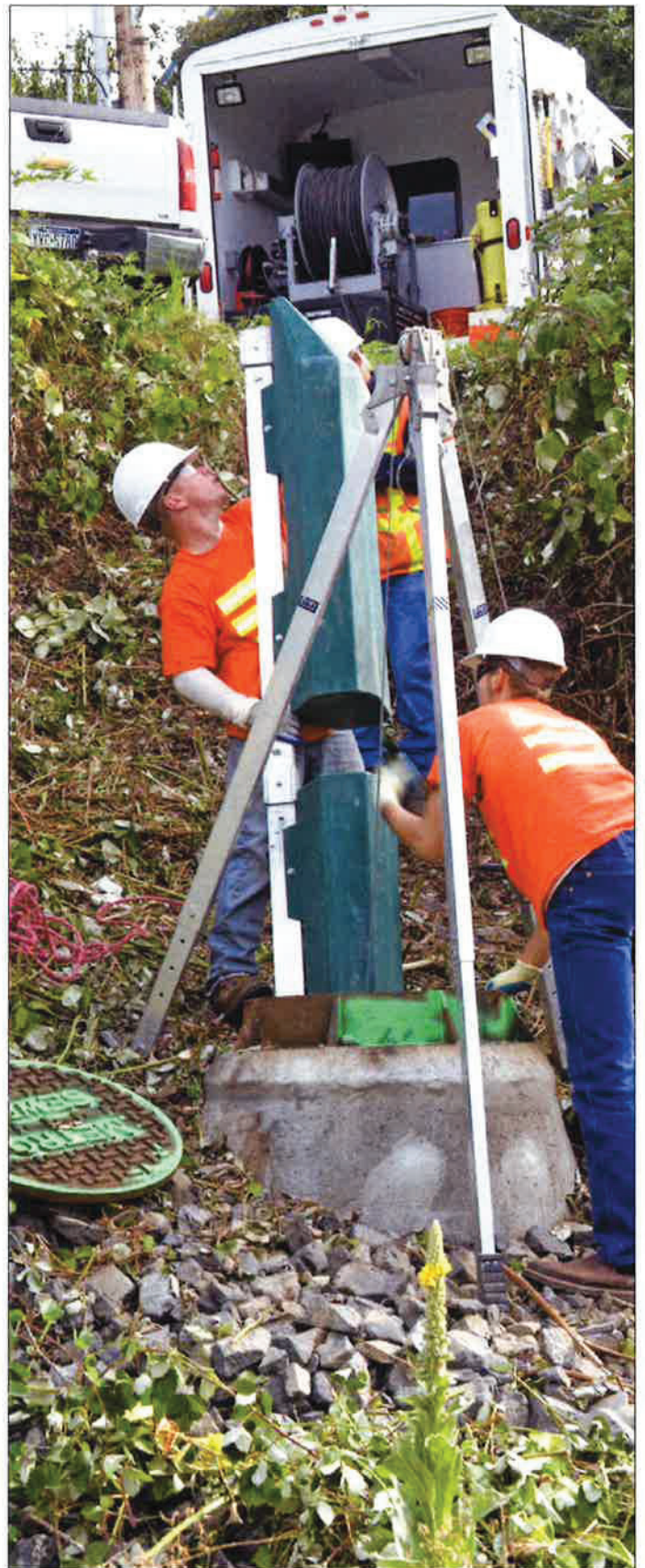
A crew from Pipe Experts Inc. of Tumwater, Wash., prepares a CCTV camera and sonar platform for the inspection of a 96-inch interceptor.
